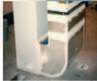
Sealed Ductwork
